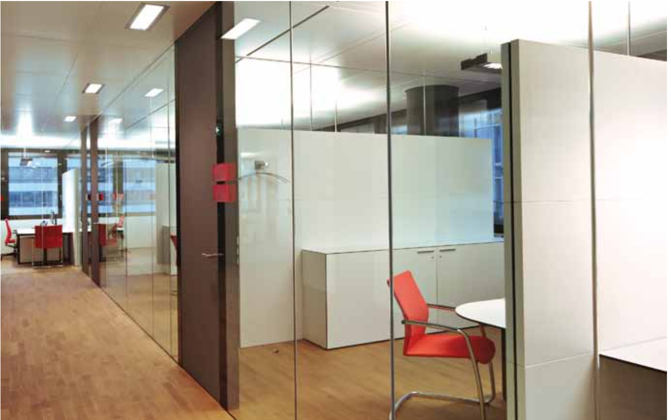
Chamber of commerce, Bolzano – Glass partition with integrated profiles into the floor and ceiling.
